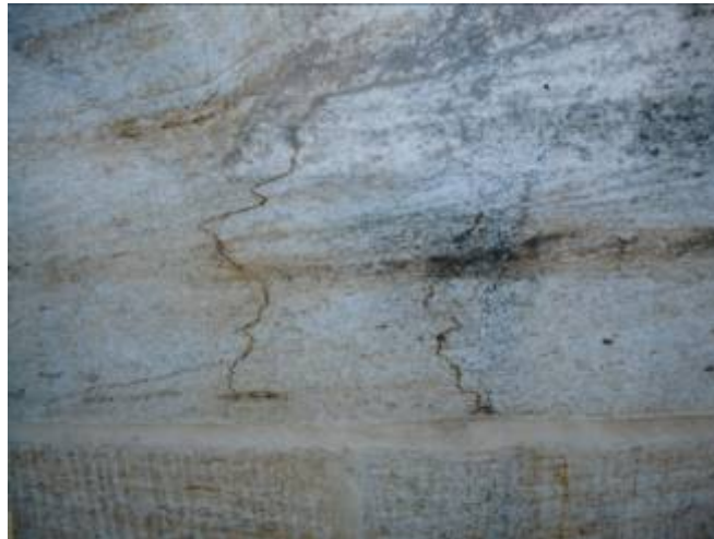
Figure 7 Pseudo-stylolites. Probably the result of small lateral displacements.
