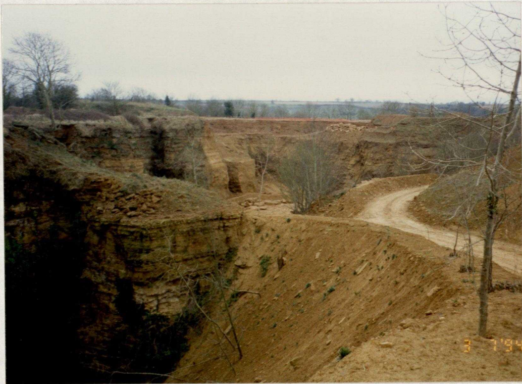
PHOTO 1. GENERAL VIEW OF LARGE WORKING QUARRY (AT SOUTHERN END OF HAM HILL) VIEWED TOWARDS THE SOUTH
